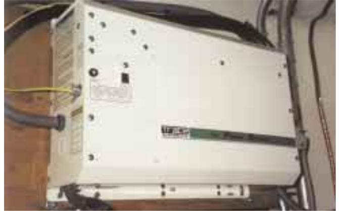
**The Trace inverter draws 5 watts when in search mode, and about 12 watts when operating.**
